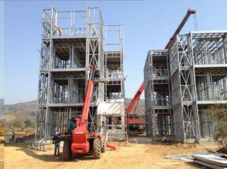
ERECTION –DIFFERENT STAGES
