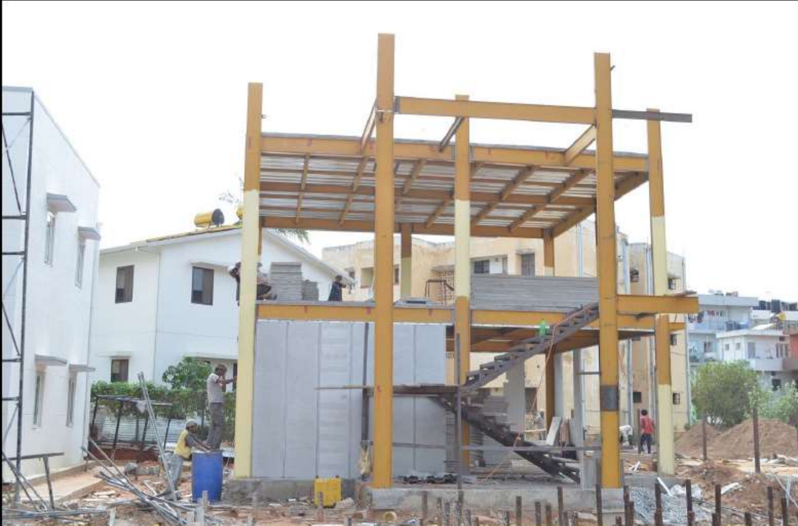
Steel skeleton with Aerocon panel infills
